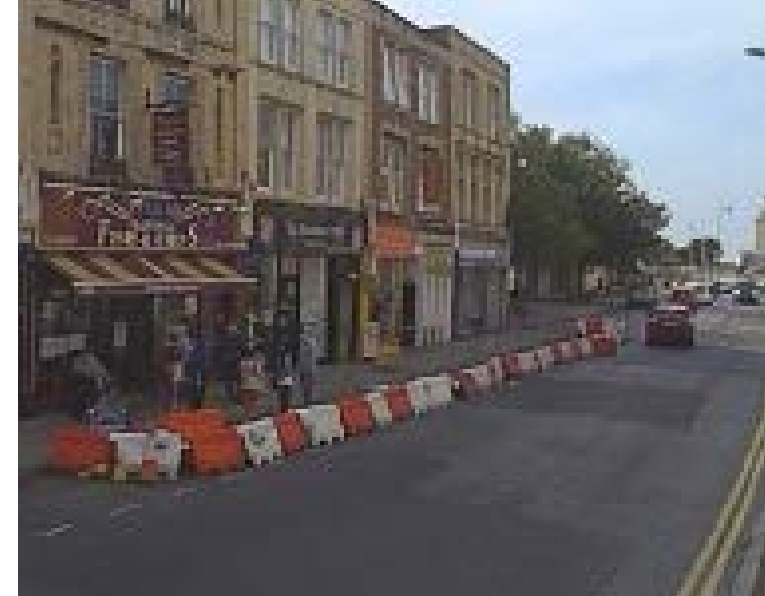
Emergency Active Travel Fund measures to support active travel and social distancing measures at busy town centre locations, such as on Waterloo Street in Weston-super-Mare
